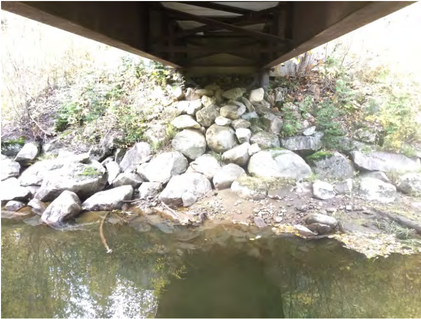
Left Bank Abutment when facing downstream
