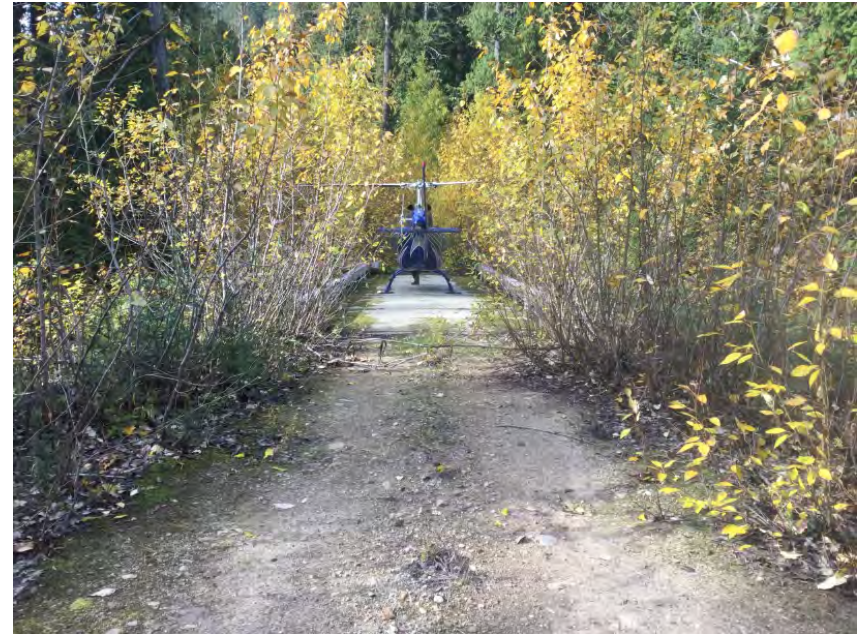
Approach from Right Bank when facing downstream
