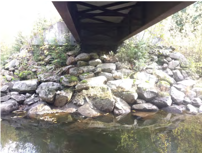
Right Bank Abutment when facing downstream
